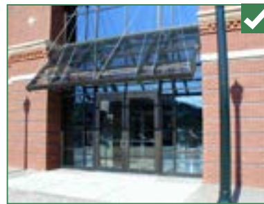
Metal and glass canopy interprets the historic role of a canvas awning or metal canopy and clarifies entry on this new building.
