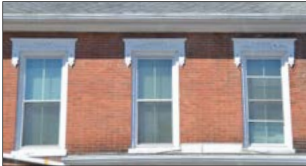
The careful design and placement of the storm windows in New Bloomfield maintains the character of the historic windows beneath.
