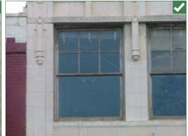
Historically, most windows installed during Perry County's primary period of downtown commercial development were 1-over-1, or 2-over-2 in pattern. However, installations such as the 6-over-1 pattern shown above were used successfully to introduce character and variety.
