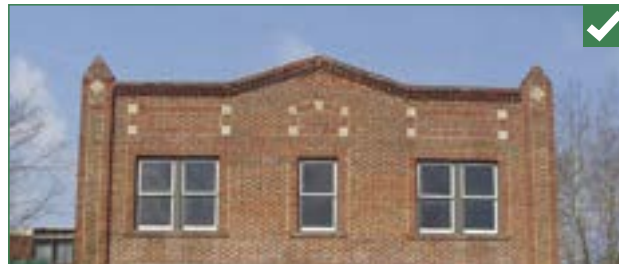
The triangular treatment at the center of the roof line creates interest and delineates entry. The upper floor details such as precast tiles and recessed panels above the windows creates interest at the second floor.
