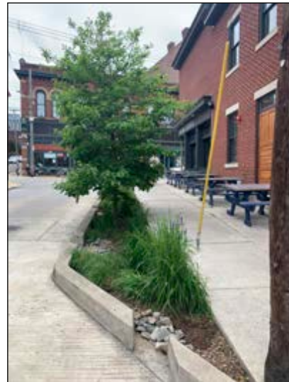
Good example of a flow through planter to filter rainwater in an attractive manner.
