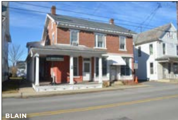
BLAIN The Library in Blain is housed within a former residence that features a gabled roof over the main structure and hipped roof over the wraparound porch.
