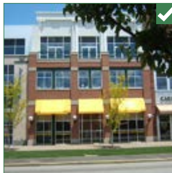
The awnings on this new commercial building are well-executed and respond to the window and doorway openings.
