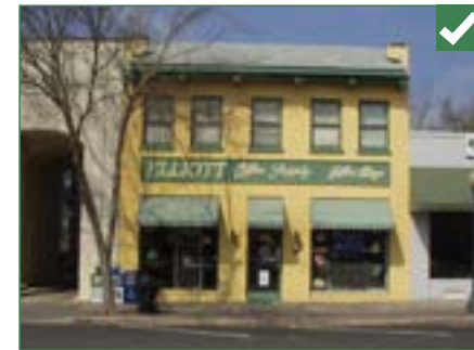
Occasional variety in the roof line is acceptable, particularly when horizontal alignment with adjacent buildings is maintained. This roof line would have been even more appealing had the original tile roof material been maintained.
