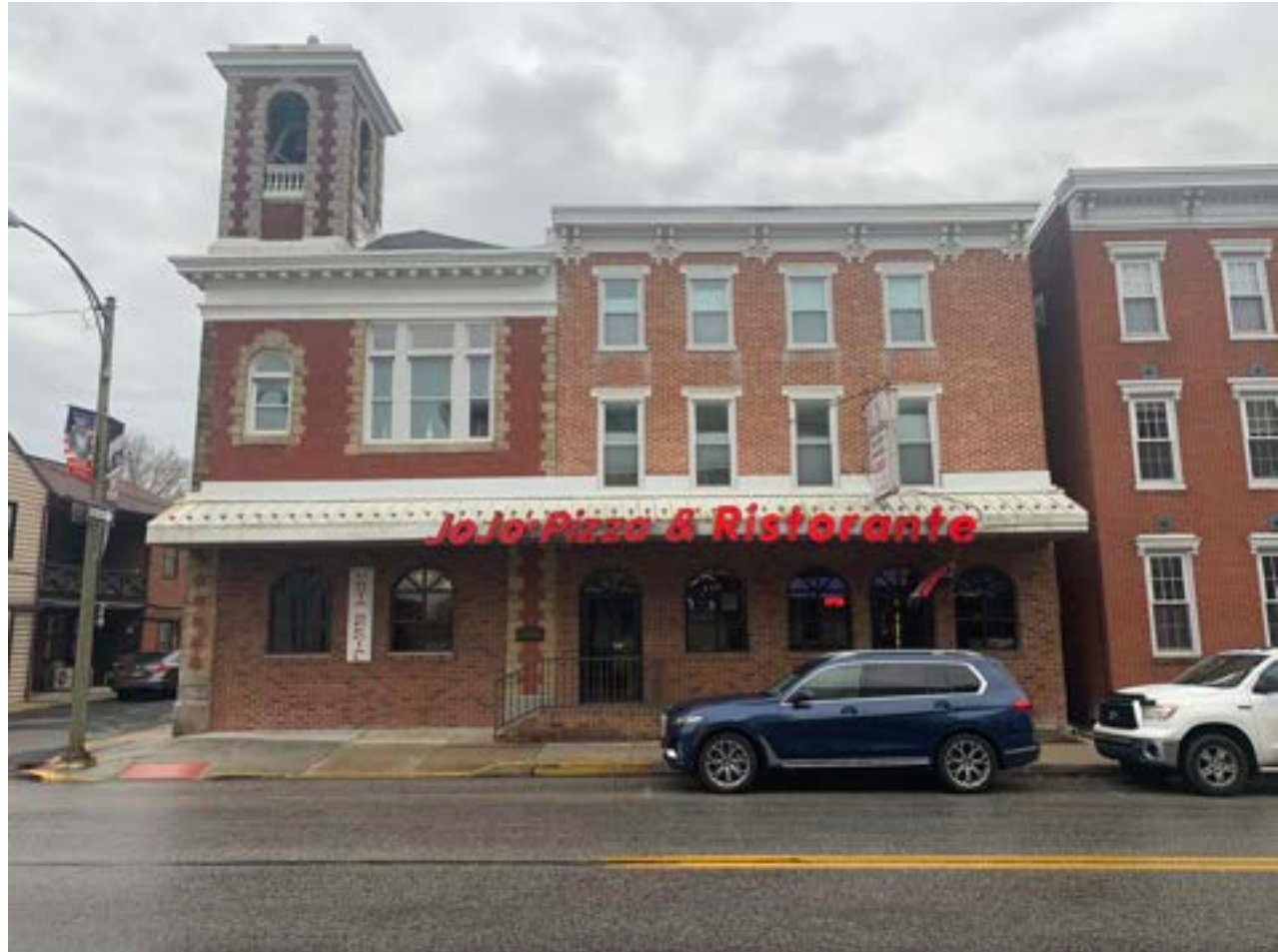
Bad example of use of smaller window that replaced original storefront windows.
