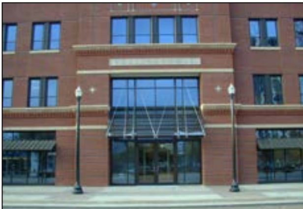
Successful “contemporary interpretation” of the traditional storefront. This building uses a glass canopy to create the covered entry of a historic storefront canvas awning.
