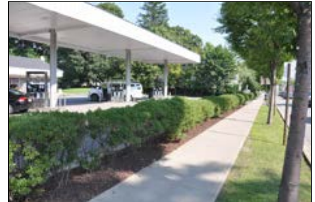
Good example of how a landscape hedge can minimize the visual impact of the large expanse of pavement associated with a gas station.
