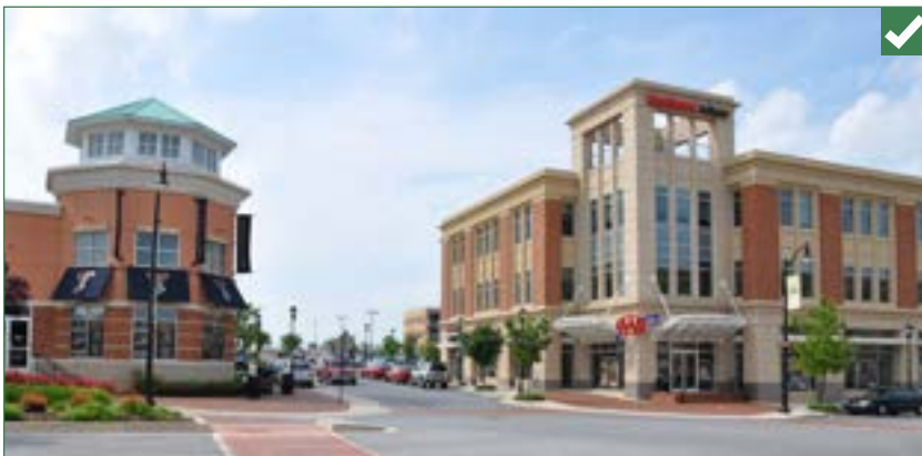
Canvas awnings (left) and metal canopies (right) on these two new commercial buildings illustrate appropriate awning treatments that respond to the windows, doors, and associated architectural forms.
