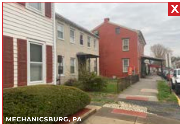
Bad example of infill development that does not respond to the setbacks of either of the adjacent buildings.
