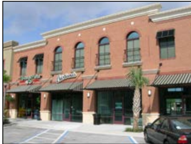
Positively, this balcony installation provides a level of detail/ornament. Negatively, it should be questioned why you would have a balcony that is inaccessible/non-functional since the windows behind are fixed in nature.
