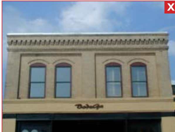
In this example, the original arched-top windows were removed and rectangular units were installed in their place with a wooden "filler" inserted in the arched area. This gives the appearance of an "eye lid" closing above the windows. Always fill the opening with an appropriately sized window.
