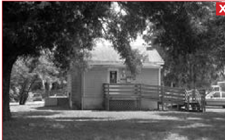
This handicapped ramp is inappropriate because it dominates the small building. The enclosure of the front porch also would not meet the Architectural Review Board guidelines.
