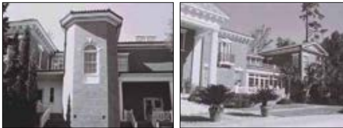
Built in the early 1900s, this residence was enlarged considerably for use as a hotel. Both rear and side additions were made for the new use. While the brick and roofing of the additions match that of the old structure, the detailing is less elaborate. The form of the original house, which is still dominant, is evident.
