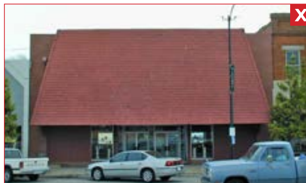
The roof form becomes the dominant element of this façade and is incompatible with its surroundings.
