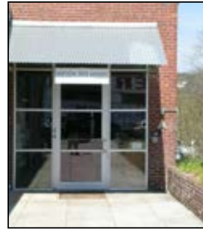
Successful “contemporary interpretation” of the traditional storefront, with three-part vertical & horizontal composition. See diagram at right.
