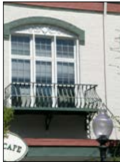
Well executed balcony and support bracket.
