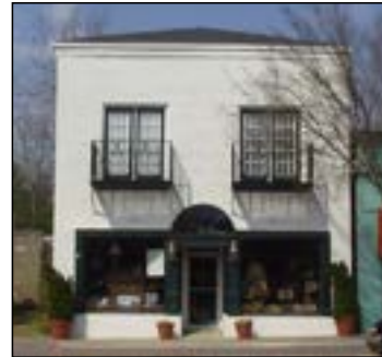
Appropriate balcony installation in Aiken, SC.
