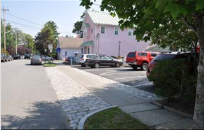
Good example of how the sidewalk treatment can extend across a parking lot apron to prioritize the pedestrian.
