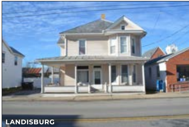
LANDISBURG This residence in Landisburg uses a combination of hip and gabled roofs.
