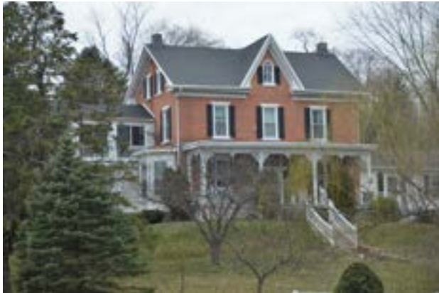
The small, one-story additions on the left do not detract from the original design of the house.
