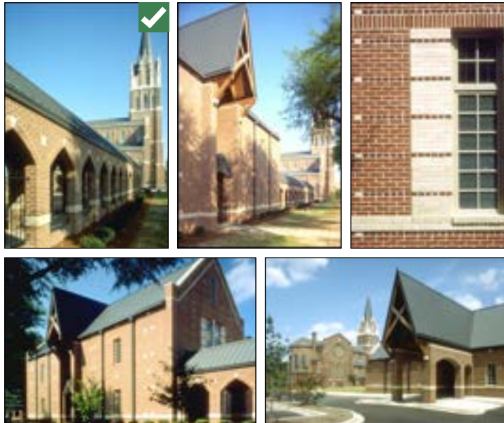
Excellent example of a historic church that built a new addition. The new addition did not pretend to be historic, but rather interpreted the historic detailing of the building (e.g., brick patterns, water table, Gothic windows, spire) in contemporary ways and with modern materials.
