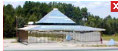
The reflective glass of this building would be highly inappropriate in a context such as Perry County where brick is the predominant building material.
