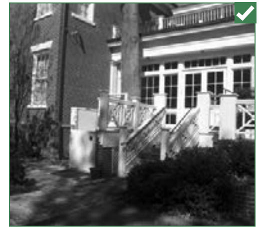
The wheelchair lift provides access near the front entrance and eliminated the need or a ramp. Such lifts are effective for three-to-ten foot changes in elevation.
