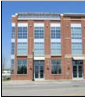
Successful “contemporary interpretation” of the traditional storefront separating the “display windows” with brick piers, and maintaining recessed door entry.
