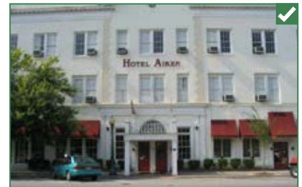
Long building sub-divided into bays with clear hierarchy and delineation of entry.
