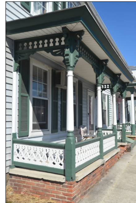
The ornate balusters and fascia of this porch provide handsome architectural detailing to the entrance.
