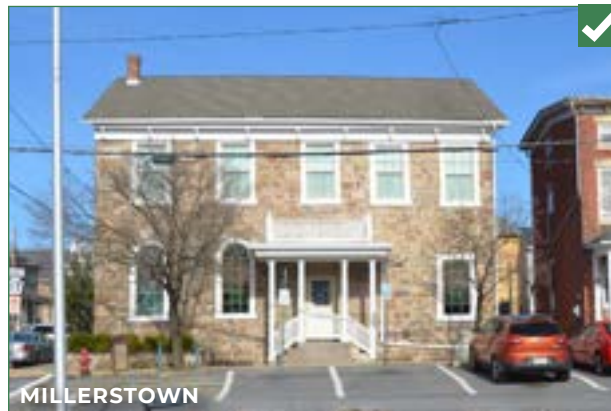
Millerstown - Stone is a common building material in Perry County.
