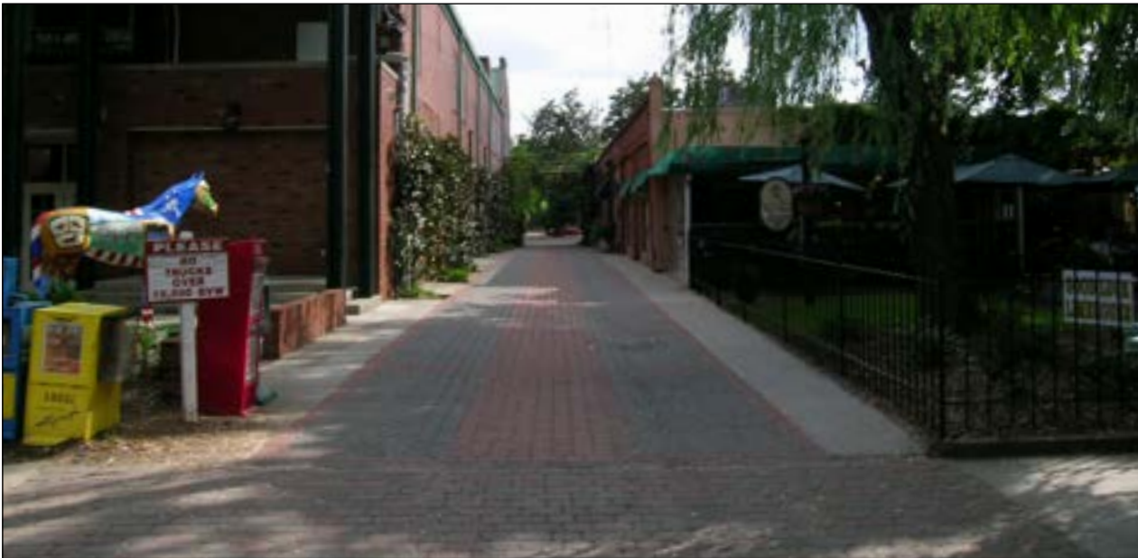
Examples of appropriate alley treatments such as pavers and sidewalks and fencing that meet the needs of both pedestrians and automobiles.
