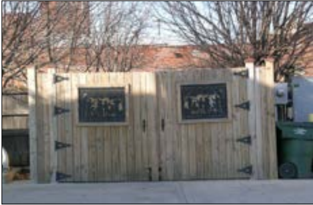
Good example of screening service equipment and trash bins utilizing wood gates with wrought iron ornament.
