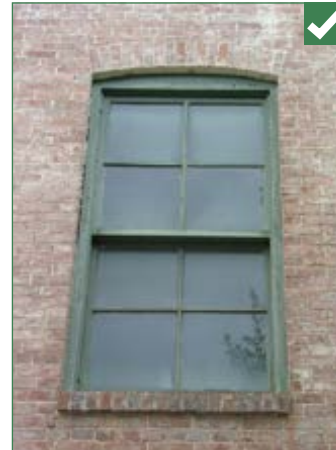
True divided light wood windows were the norm in traditional construction.
