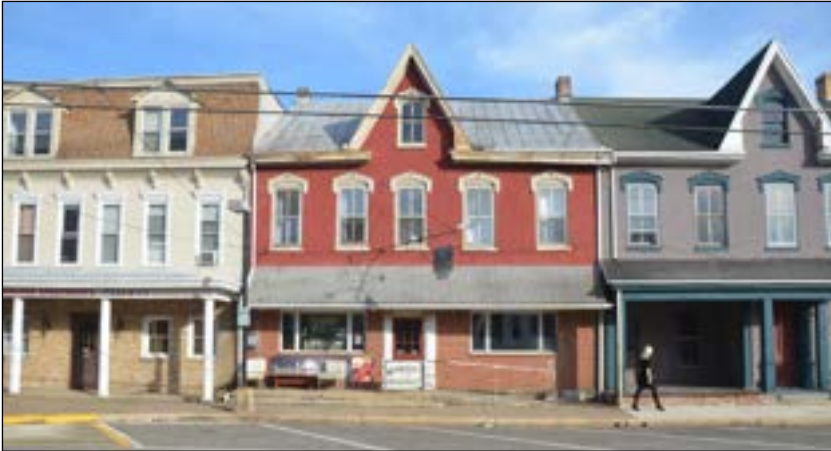
The preservation of original window in their original shape and placement, coupled with tastefully applied storm windows on this row of residential form buildings in Duncannon creates a harmonious appearance in their downtown district.
